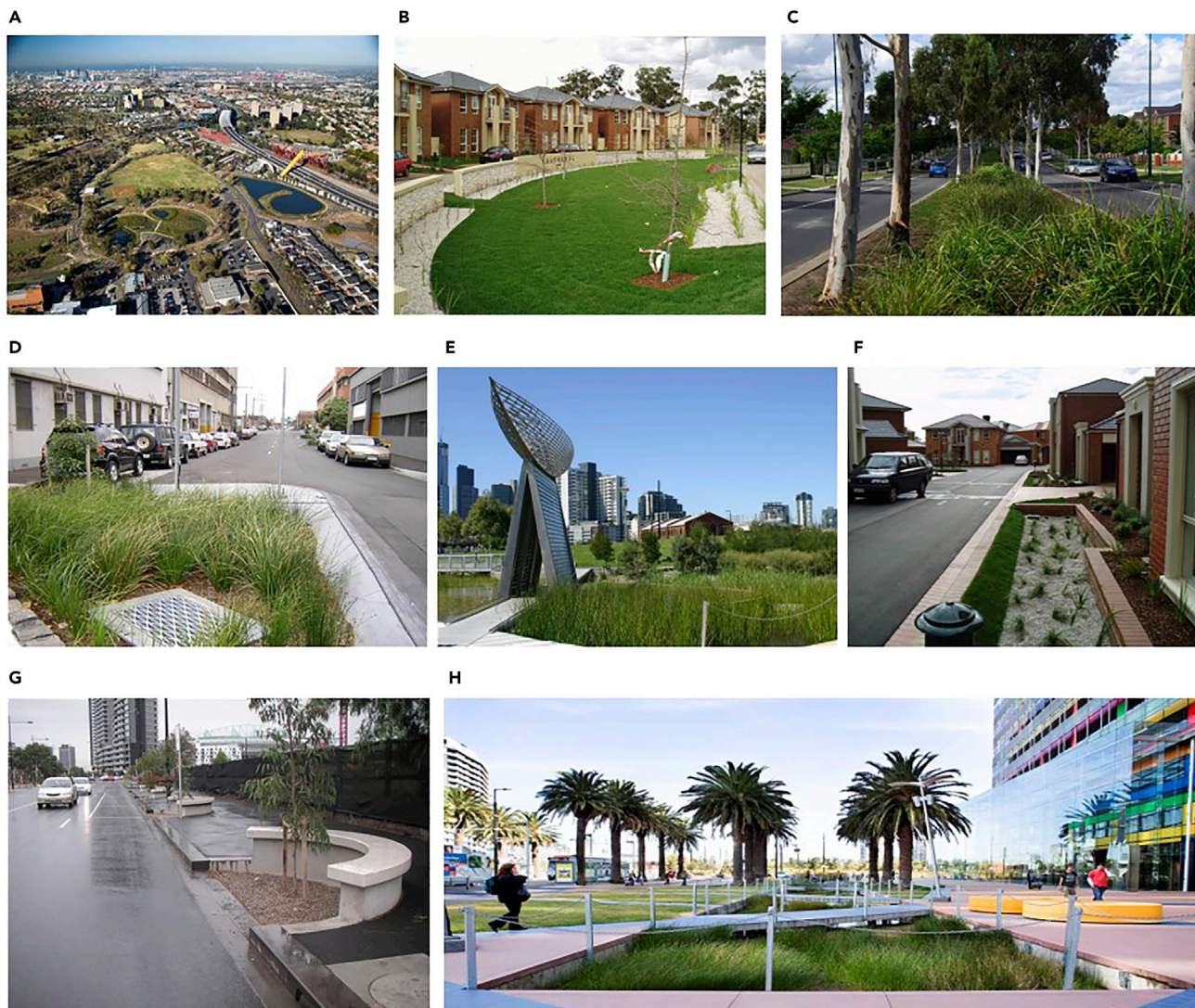
Figure 2. Various Scales of Stormwater Bioretention Systems Constructed in Melbourne, Australia
