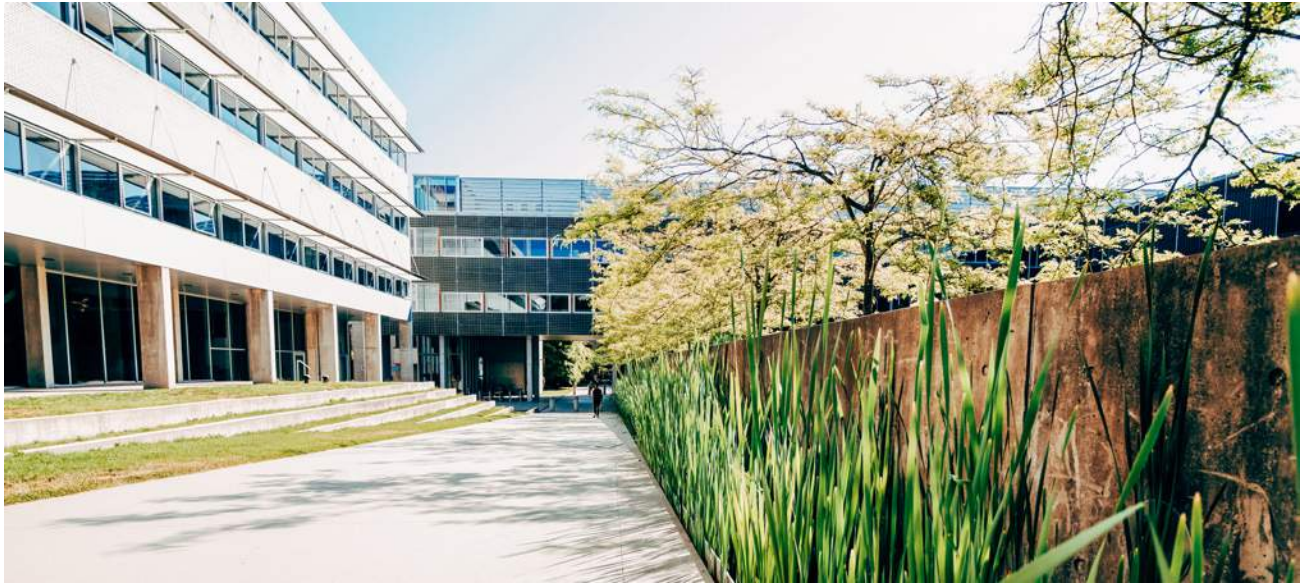
..... Bioswale at the Beaty Biodiversity Centre improves the quality of rainwater runoff ..... PHOTOGRAPHER: PHILIP BERTOGG
