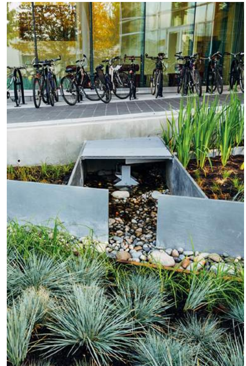
UBC CIRS Building rainwater infiltration system PHOTOGRAPHER: DON ERHARDT
