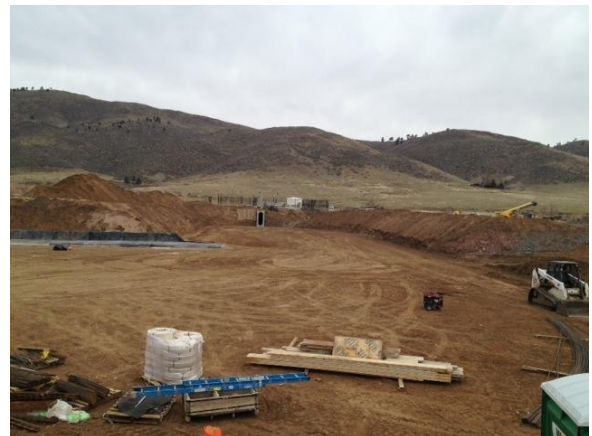
Construction of Pre-Sedimentation Basin, March 2013
